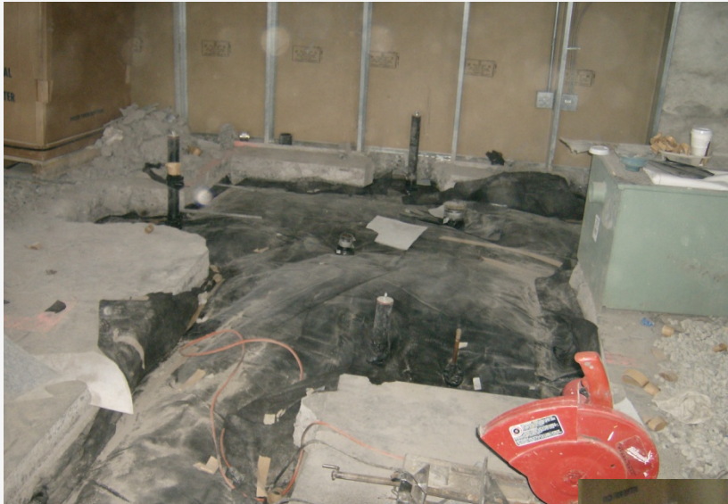
Liner Repair and Testing
