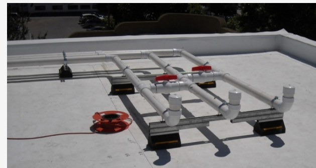
Piping, but no fan on roof
