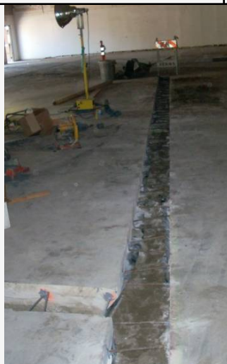
Sub-slab trenching for vent pipe
