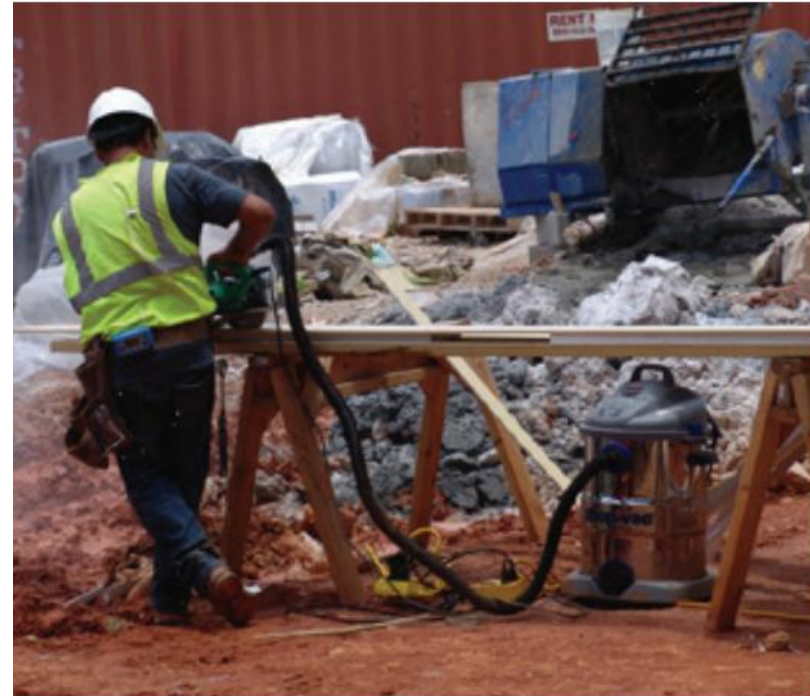
Worker cutting fiber-cement board outdoors using a handheld power saw and dust collection system. The dust collection system consists of the shroud on the saw, hose, and dust collector positioned between the saw horses.
